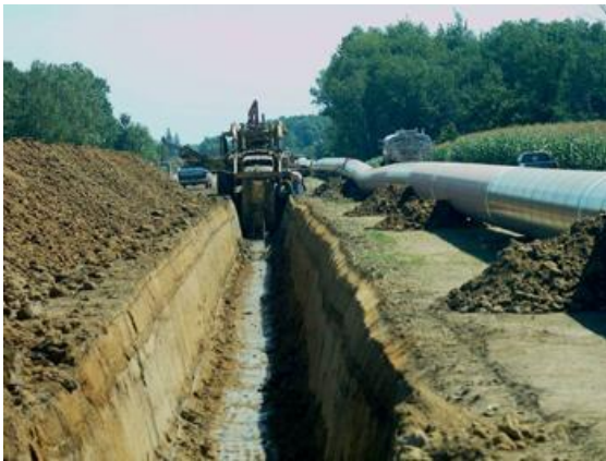
Dawn to Parkway/Kirkwall Pipeline
